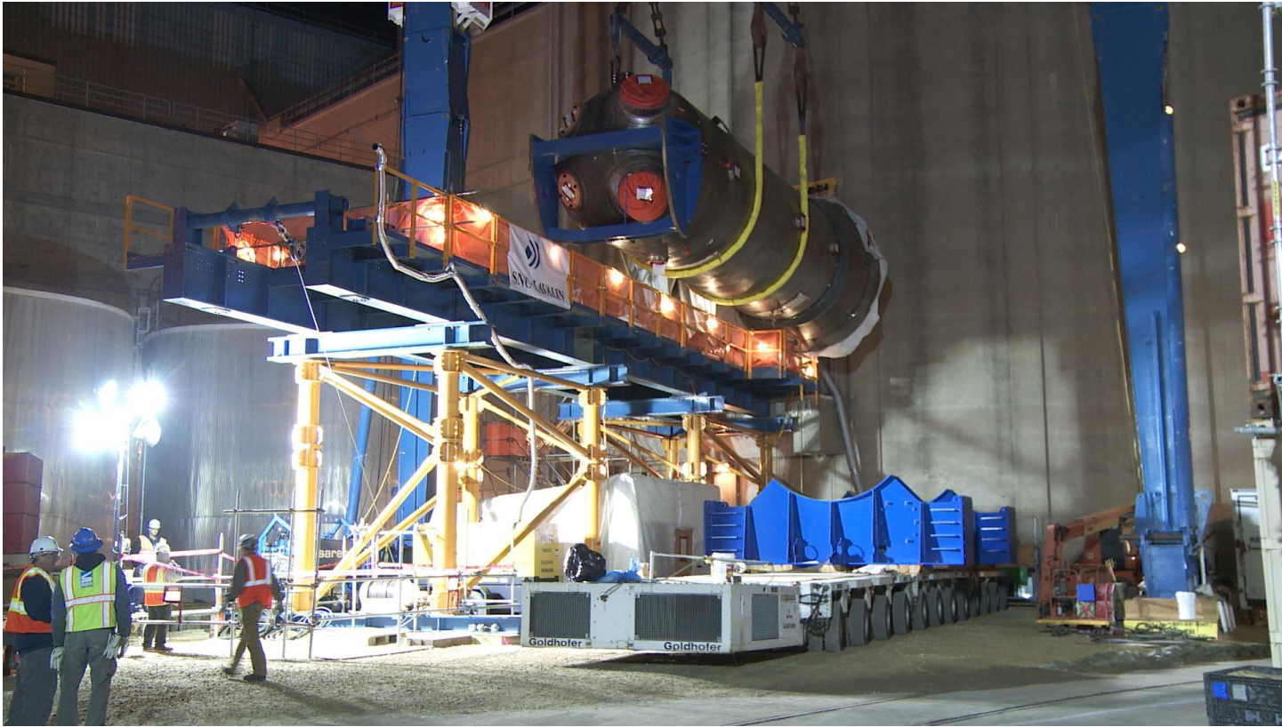
Recambio del Generador de Vapor de Prairie Island NPP, circa 2014 (1973-active)
